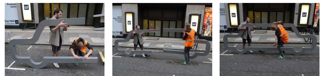
**Step 1**: Slide top and bottom connecting member into one half of the car bike port. Secure using M10 Torx bolts. Make sure the correct slots are inserted facing the right way. The bottom member must insert with the two side bolt holes on the same side as on the car bike rack.
