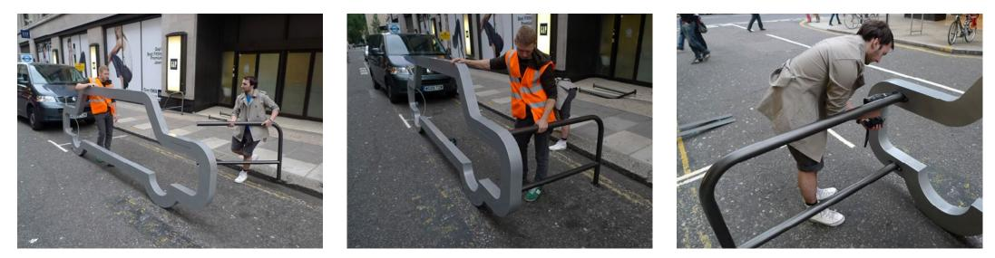
Step 3: Take a side rack and place it, lining up the drilled holes. Place 4 x M8 Torx bolt into holes and screw into place using electric drill on low speed. Repeat on the other side.
