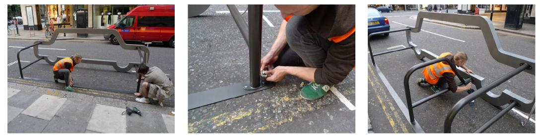
Step 4: Take the steel floor plate and place it under the metal rack, lining up the drilled holes. Screw the short M8 Torx bolts into plate. If the holes do not line up, loosen the Torx bolts in the car frame until the holes line up before retightening.
